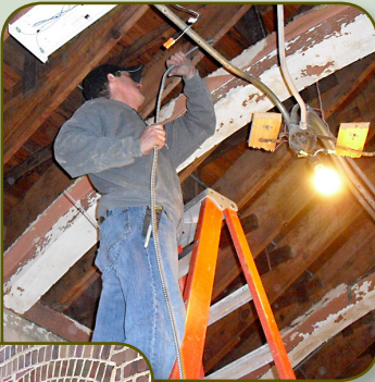
ABOVE: Jason Rhodes of Seward Electric runs wire above ceiling beam for lighting in the lobby.
