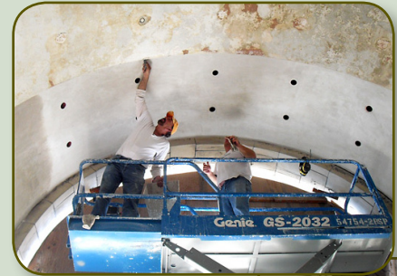
ABOVE: Perfection was the order of the day as the crews worked together to bring back the magnificence of the barrel ceiling.
