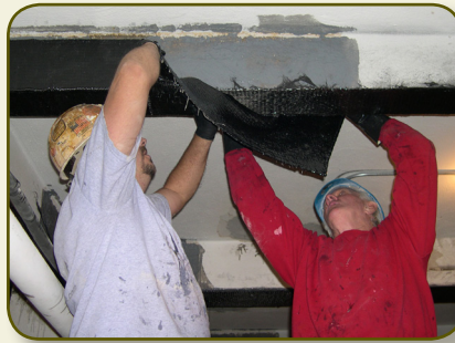
Contractors applying epoxy soaked FRP to Colonial Fox basement beams.
