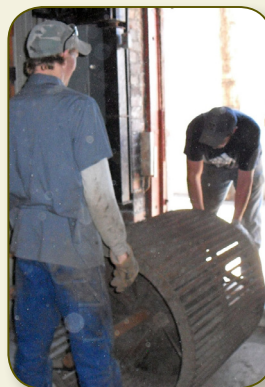
ABOVE: SEK Heat & Air takes apart the air duct high above the stage, behind the proscenium arch.
